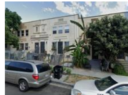
Columbia Place, West Lake Source: Google Earth
