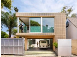
Address unknown, Venice Source: bau10 architecture
